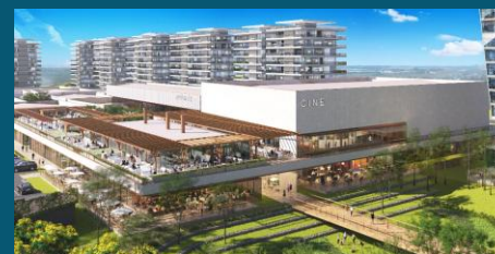
"Distrito Diagonal" (La Plata – BA Prov.) Ongoing development +22,000 sqm
